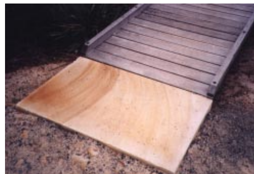
Combination of sandstone, timber and gravel pavements
