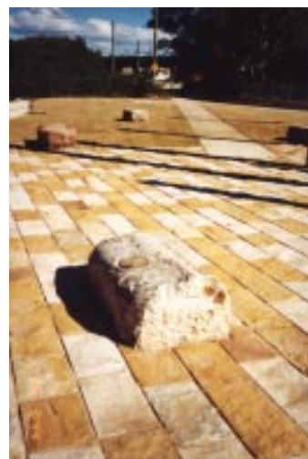
Sandstone paving types and patterns, used to other pedestrian thresholds in Shepherds Bay. should be reflected in the design of the depot site
