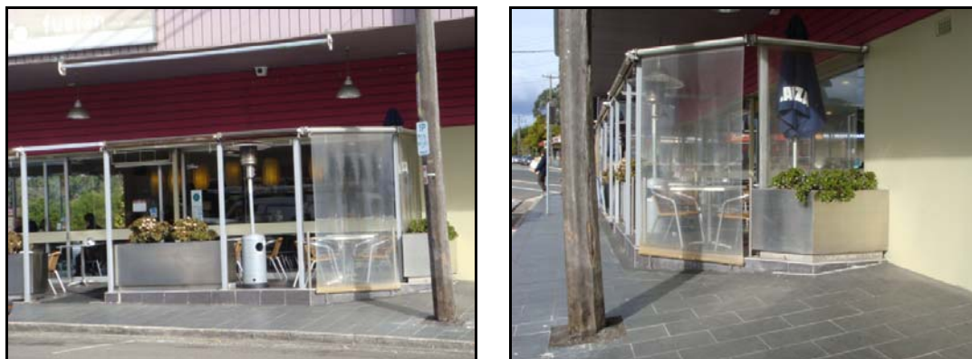
Figure 2 Example of minor works to the footpath area ensuring a level platform for the outdoor dining area. Diners are protected from the change in level by trellis balustrading and planter boxes.
