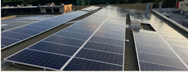
Solar panels on the roof of North Ryde Library.
