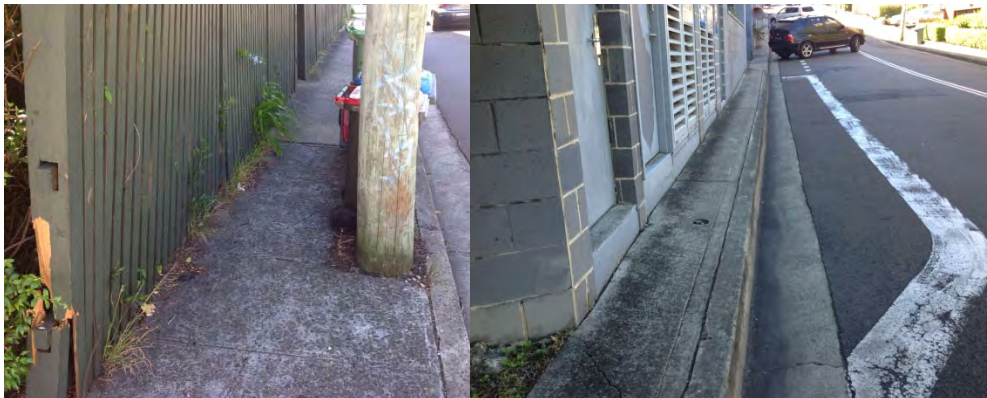
Photograph 32 Existing Footpath Deficiencies, Flagstaff Street
