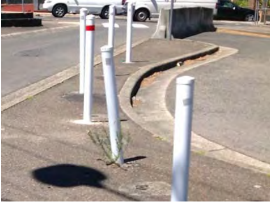
Photograph 8: Wharf Road/Meriton Street
