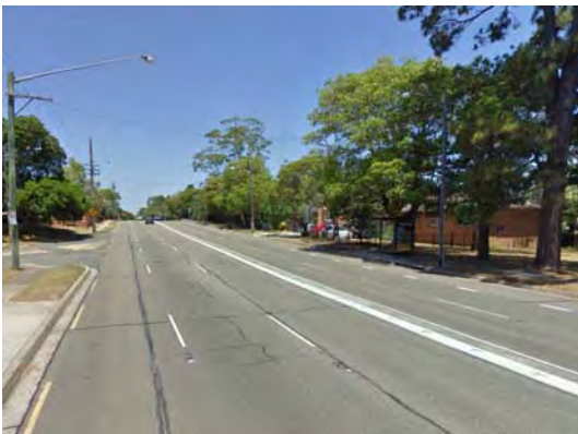
Photograph 29: Victoria Road, near Salter Street
