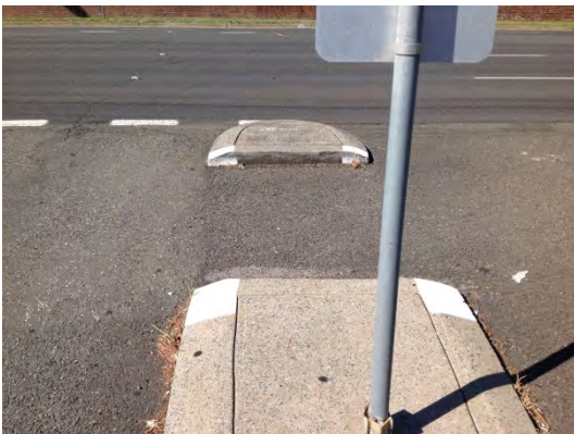
Photograph 25: Manning Road, north of Victoria Road intersection
