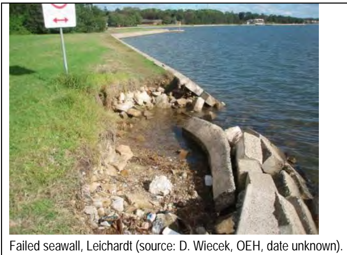
Figure 2.16: Example of Failed Seawalls
