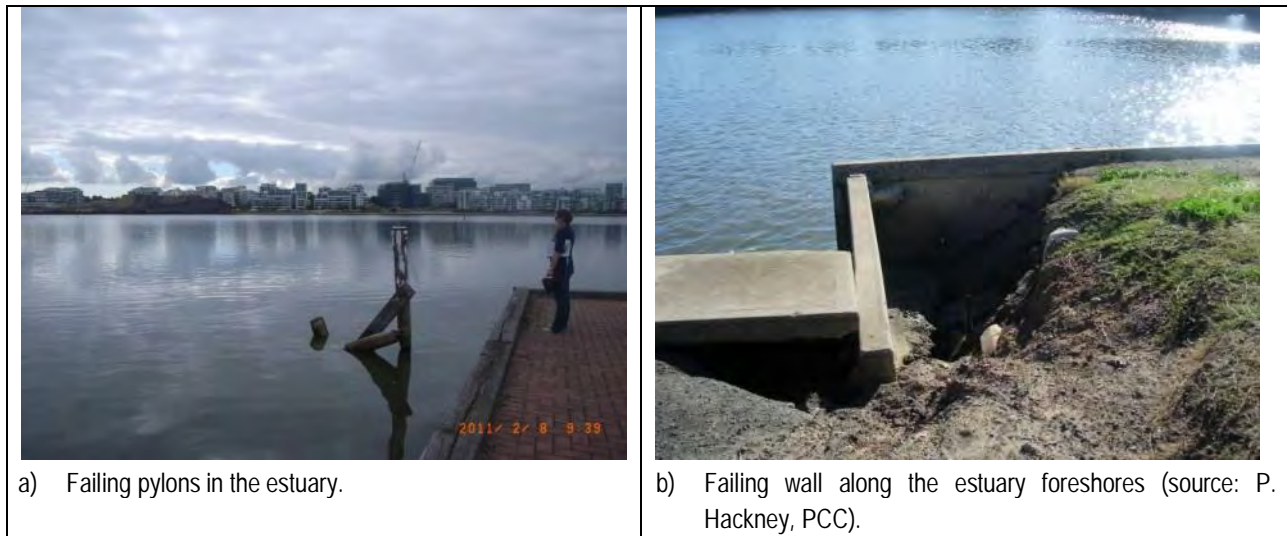
Figure 2.30: Failing Foreshore Infrastructure
