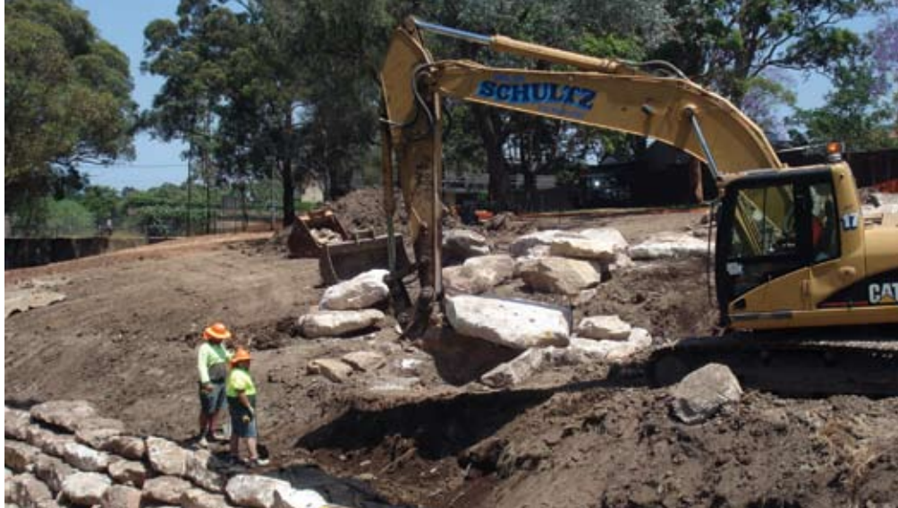
Archers Creek Restoration before (top) and after (bottom)
