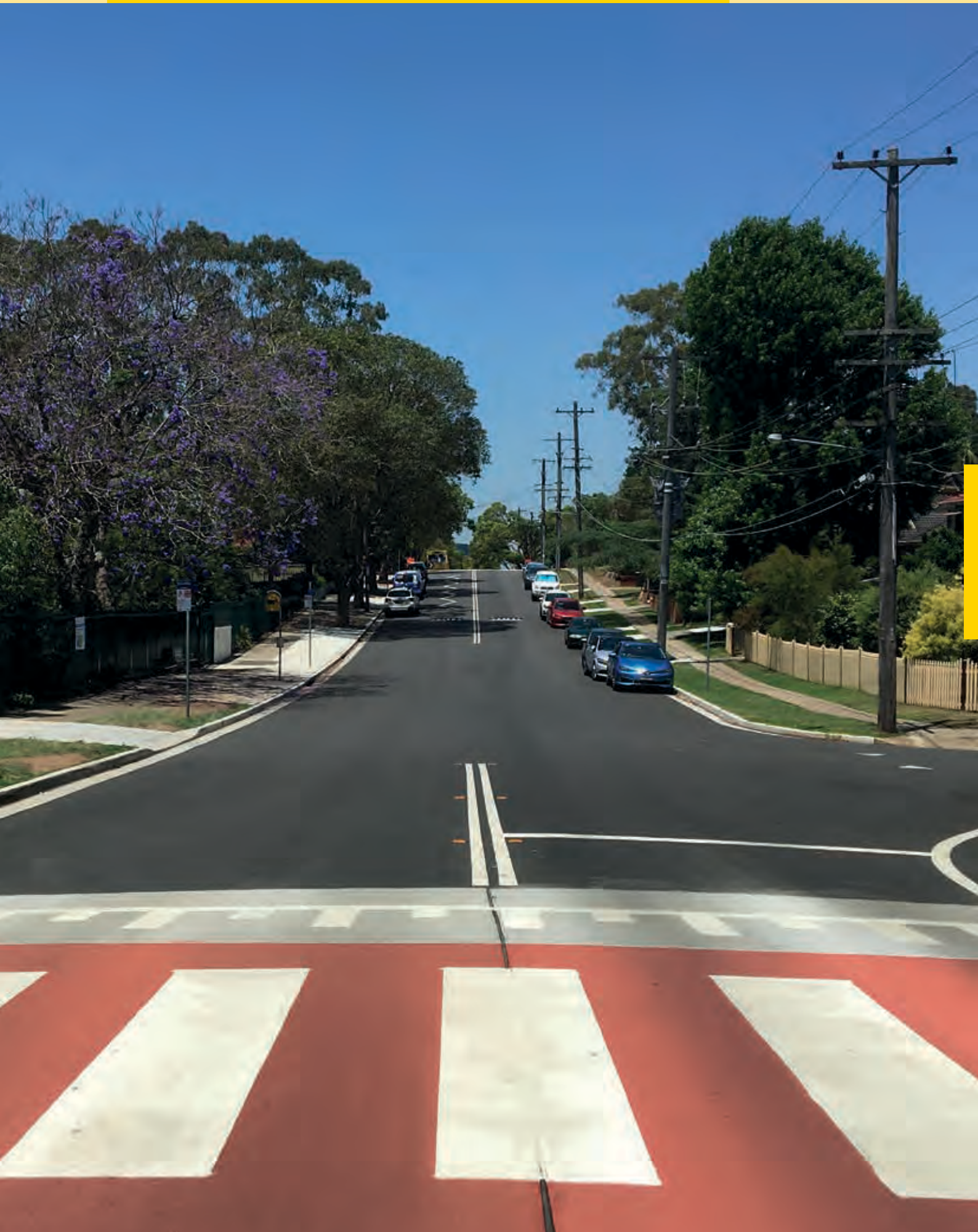
Winbourne Street upgrade West Ryde
