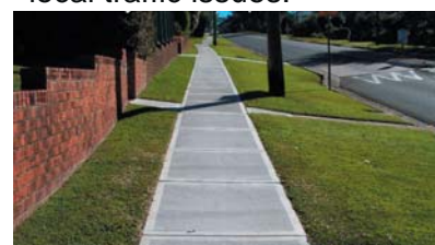
Shaftsbury Road Footpath, Eastwood
