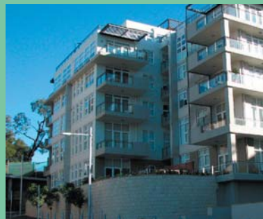
Faraday Road, Meadowbank Residential development to west of site
