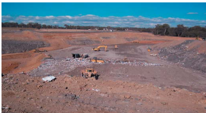
Eastern Creek Landfill
