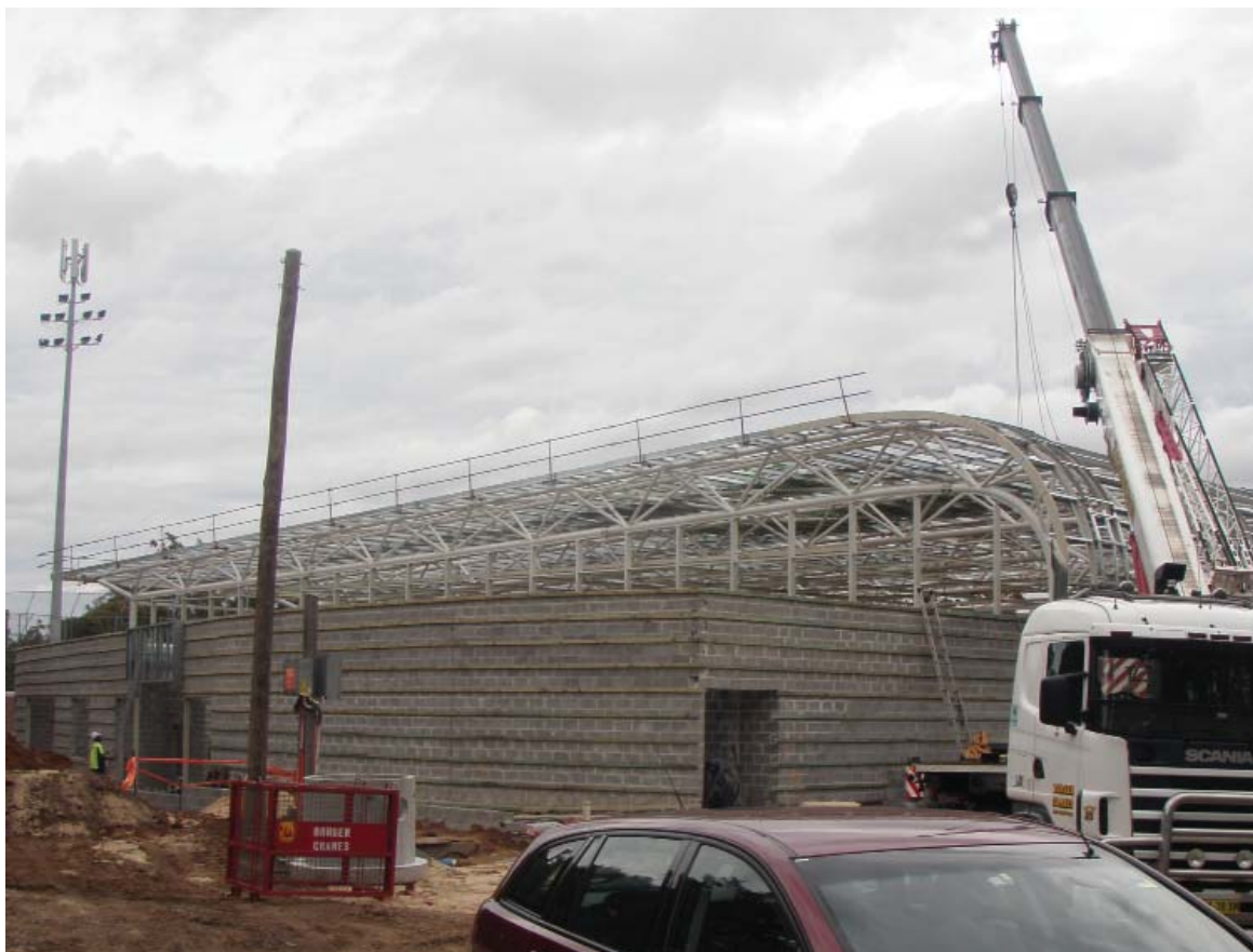
Opposite: Construction underway at Simla Road, Denistone as part of our 'Missing Links' stormwater management program Above: The Ryde Community and Sports Centre at ELS Hall Park is taking shape
