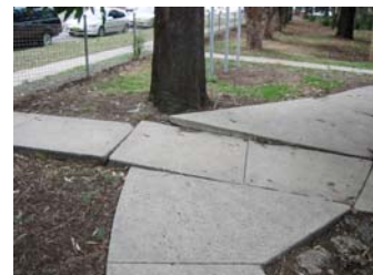
There are significant trip hazards throughout the Park from misaligned paths and tree roots.
