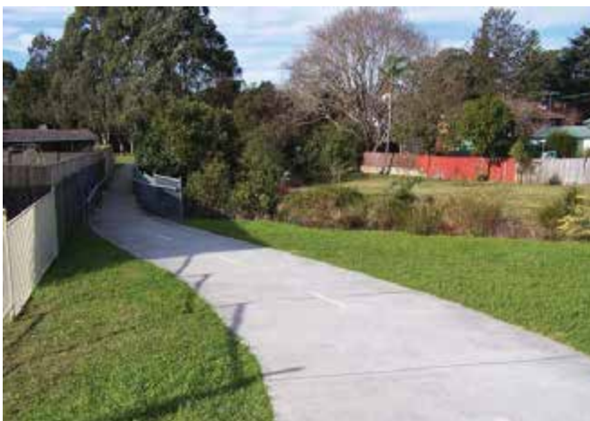
Photograph 2.3 Flinders Park entry from Bridge Rd
