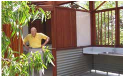
Public Toilets, Open Visibility
