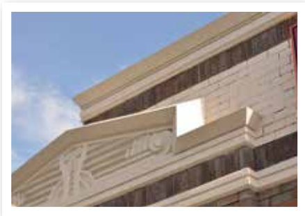
Art Deco influenced detailing to the parapet wall.
