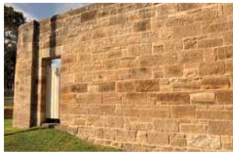
View of the stone wall.
