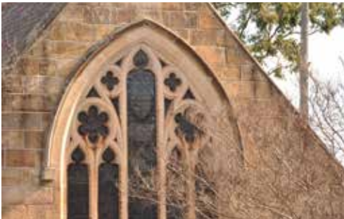
View of the main front leadlight window.
