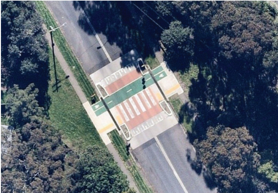
(Figure 37) Example of a raised zebra crossing with bicycle lanes on Buffalo Road. Source: Nearmap, August 2021.
