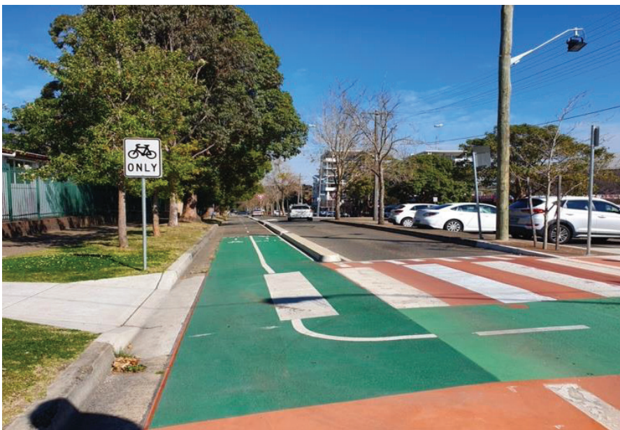
(Figure 38) Example bicycle crossing linking into a separated on-road bicycle facility, Sutherland. Source: CrossleyTP.
