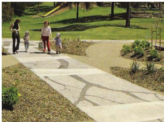
Detail Concrete Treatment Colour and texture to in-situ concrete along interpretive pathway.
