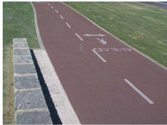
Asphalt Pavement Coloured asphalt cycleway with concrete edging and line marking (Swan River Perth).
