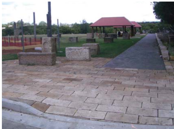
Unit Pavement Sandstone pavement to define threshold to secondary pathway.
