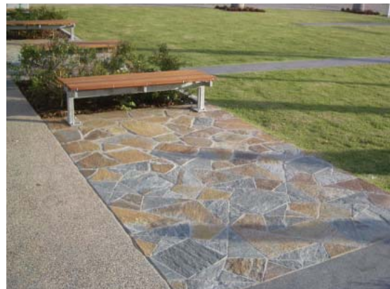
Unit Pavement Porphyry stone pavement to define separation of seating area off the recreation pathway.
