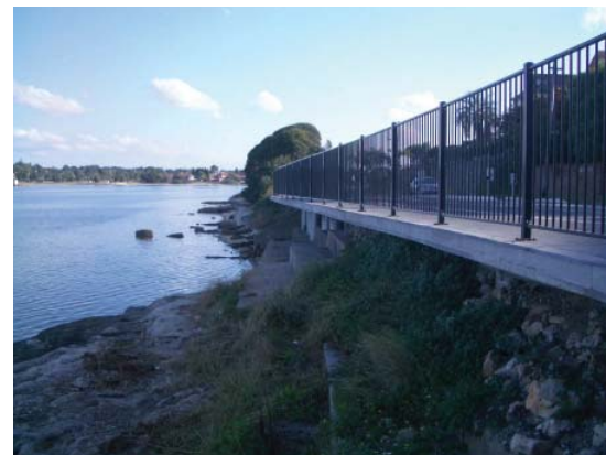
Suspended Concrete Pavement Concrete pavement elevated on pier footings to maintain level of footpath in an area otherwise restricted due to embankment (Canada Bay Trail).
