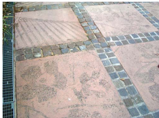
Detail Concrete Treatment Colour and texture to in-situ concrete with shot blast patterns for habitat based artworks (Roma St Parklands Brisbane).
