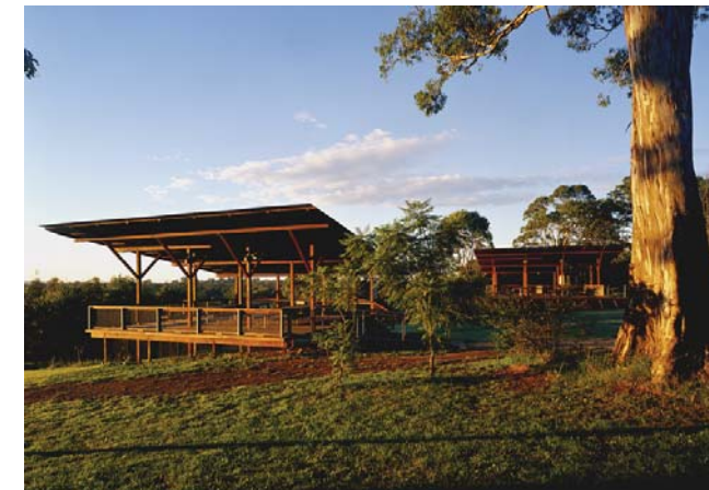
Rest shelter Rouse Hill Regional Park (Phillips Marler) Generous pavilions with BBQs and seating for large groups. Simple open style in character with park setting.
