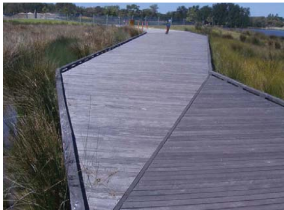
Timber Boardwalk Elevated boardwalk through rehabilitated wetland environment (Swan River Perth).
