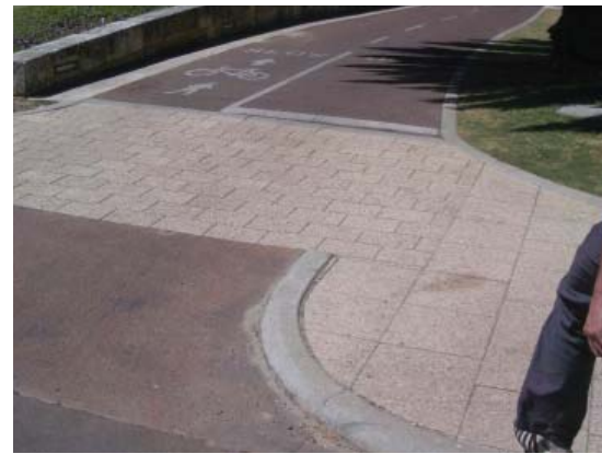
Unit Pavement Concrete unit pavement used to define threshold to car park and high use pedestrian area (Swan River Perth).
