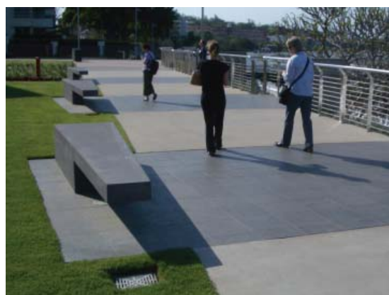
Custom Seating Custom concrete seats integrated to colour, pavement and form of the riverside promenade (New Farm Waterfront, Brisbane River)
