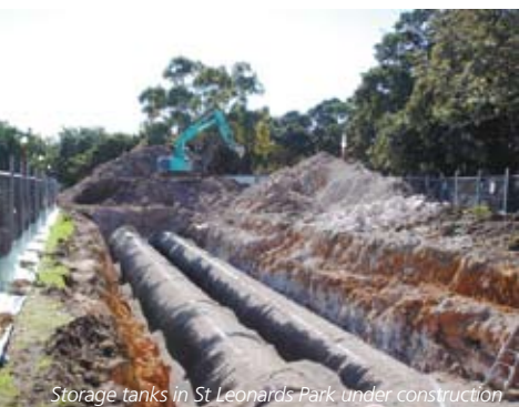
Storage tanks in St Leonards Park under construction
