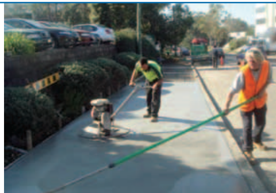
Two new shared user paths, for pedestrians and cyclists, are being constructed in North Ryde
