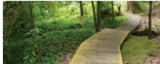
Boardwalk in the southern end of Greendale Park before the project
