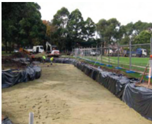
Placement of transition layer over drainage layer - 25 May 2009
