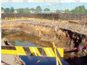
Site during remediation, showing underground storage tank pit
