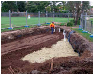
Placement of filter media over transition layer - 27 May 2009
