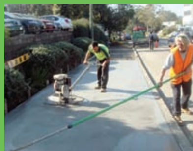
Figure 5: Two new shared user paths, for pedestrians and cyclists, are being constructed in North Ryde
