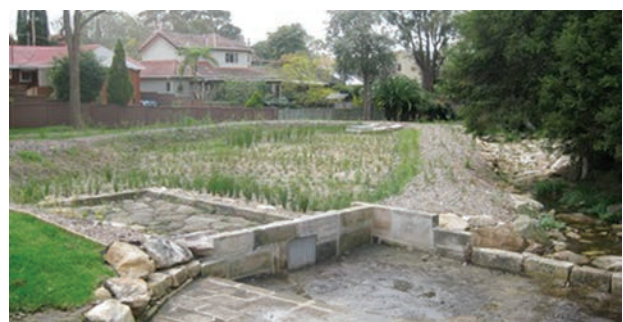
The completed bio-retention basin.
