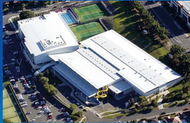
Aerial view of the Ryde Aquatic and Leisure Centre Building Complex
