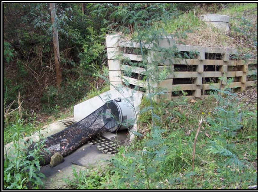
Additional Storm Trap Device installed to supplement the existing Humeceptor at Brush Farm Park
