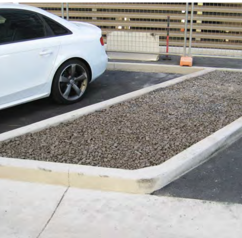
This parking space in Victoria Park has been reserved for tree planting. The tree hole is filled with structural soil (shown) and the tree hole will be excavated for better soil. The structural soil extends under the bitumen adjacent in the car space. This is a minimum soil volume required for a small to medium sized tree, in this case a Syzygium tiernianum .
