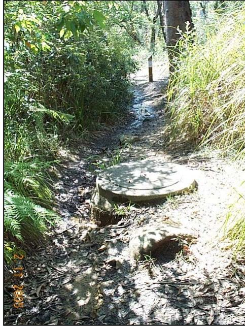
Figure 10: Leaking pipe along walking track to Terrys Ck site.
