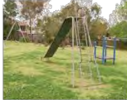
Playground without soft fall material. Unshaded site. Equipment is old, rusty and inappropriate to sustain the interest of the modern child. It should be replaced.
