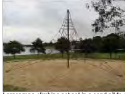
Larger rope climbing net set in a sand pit to act as soft fall layer
