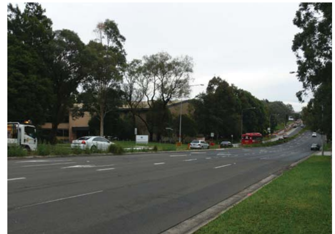
Waterloo Road has the potential to become the main spine through Macquarie Park and will help create a distinct sense of place.
