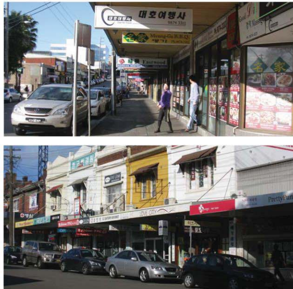
Top : Rowe Street -Existing footpath, shop front, awning relationship; Bottom: Traditional shop front buildings.
