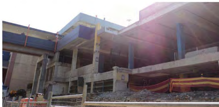
Photograph No. 2: Pedestrian Bridge Demolition Complete
