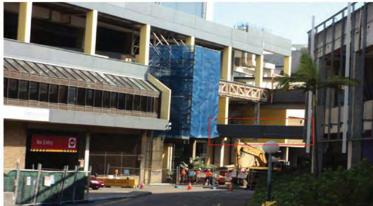
Photograph No.1: Pedestrian Bridge (pre demolition)
