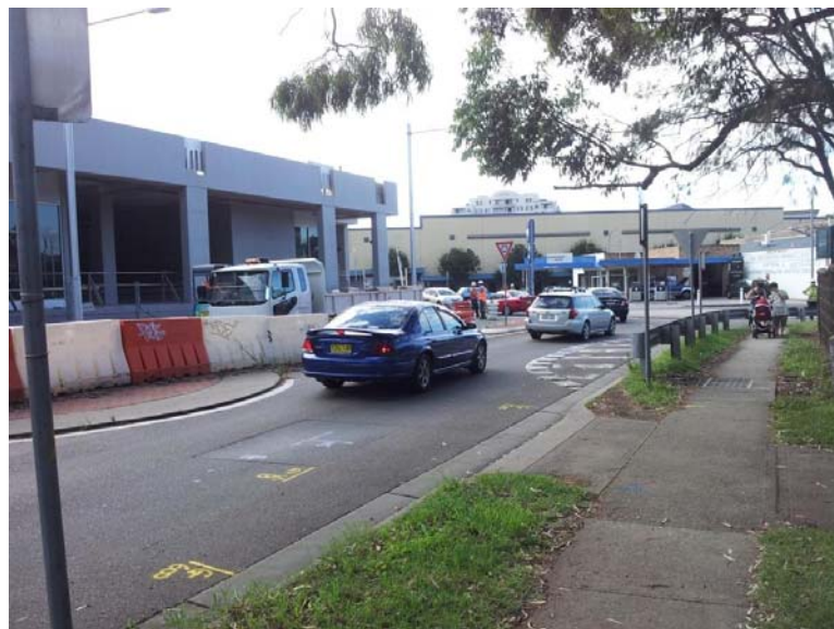
Figure 1: Roadworks commenced on Chatham Road, West Ryde date 11 March 2013
