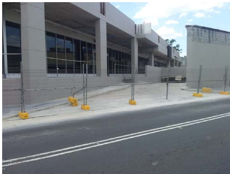
Figure 3: Single entry and exit location on New Market Street, West Ryde
