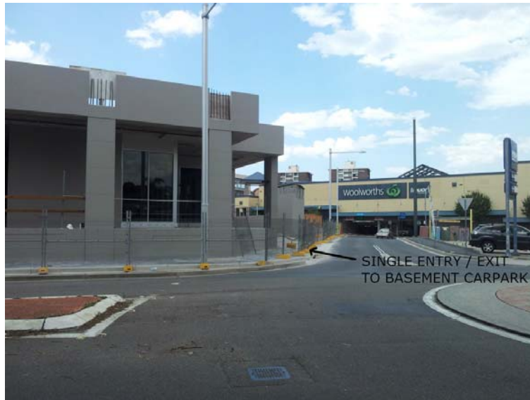
Figure 2: Single entry and exit location on New Market Street, West Ryde
