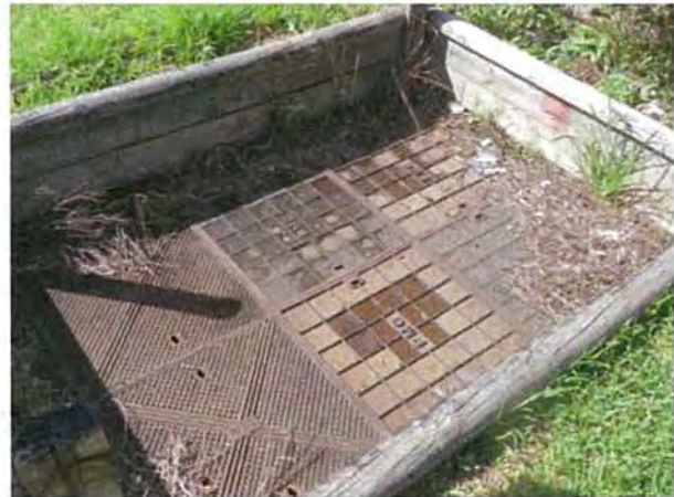
6. Unidentified services pit, PMC manhole covers (facing north).
