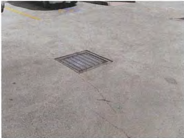
5. Minor cracking around stormwater drains (facing north).
