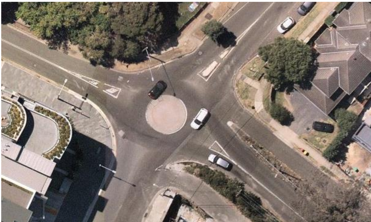
Figure 1: Existing Roundabout Intersection of Constitution Road and Bowden Street
