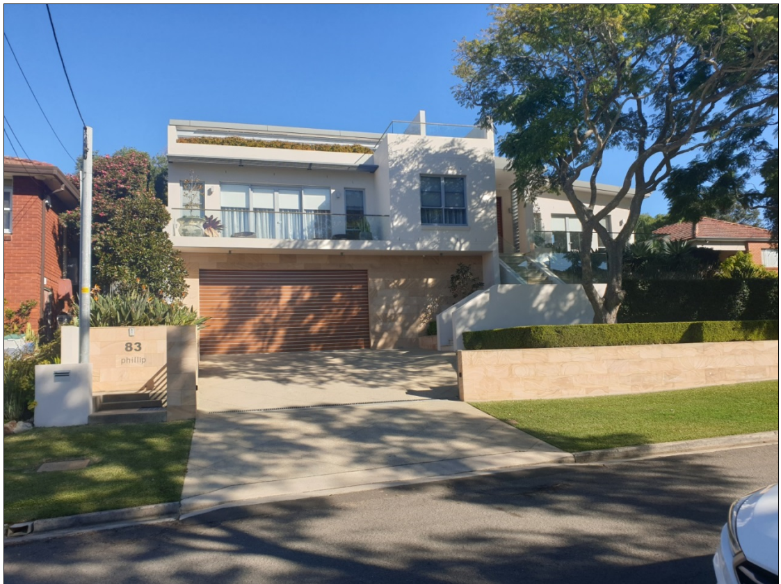
Figure 1 - The site as viewed from Phillip Road
