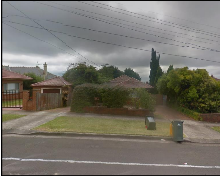
Figure 6: Single storey dwelling located at 32 Darvall Road (to the rear of the subject site)
