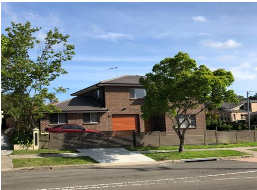
Figure 6 – 36 Clanalpine Street, as viewed from the northern (i.e. opposite) side of Clanalpine Street. Source: CPS – Site Inspection, 16 October 2018
