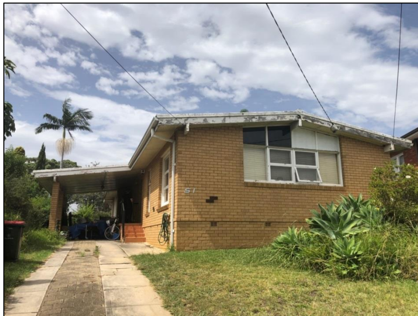
Figure 5: Adjoining property to south, No. 51 Lavarack Street.
