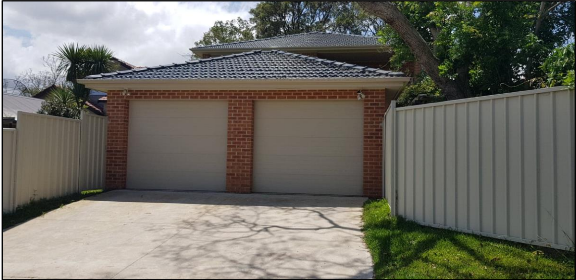
Figure 8: Vehicular access to 6 and 6A Norma Avenue.
