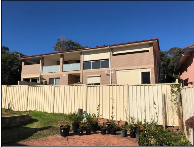
Figure 7 Western elevation of existing dual occupancy at No. 205 Vimiera Road
