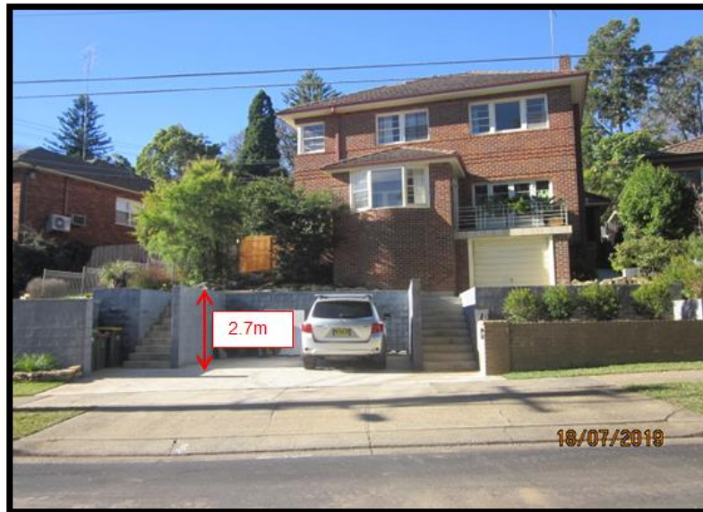
Figure 8: The existing dwelling and proposed carport. This photograph demonstrates that part of the approved garage has been constructed in accordance with the original development consent. Figures 9 & 10 show the approved garage and the proposed carport. The amended proposal results in a significantly less imposing structure than the previously approved garage.
