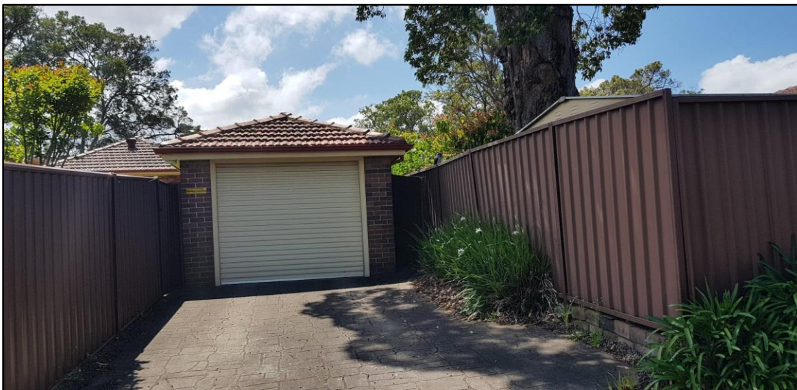
Figure 9: Vehicular access to 8 Norma Avenue.
