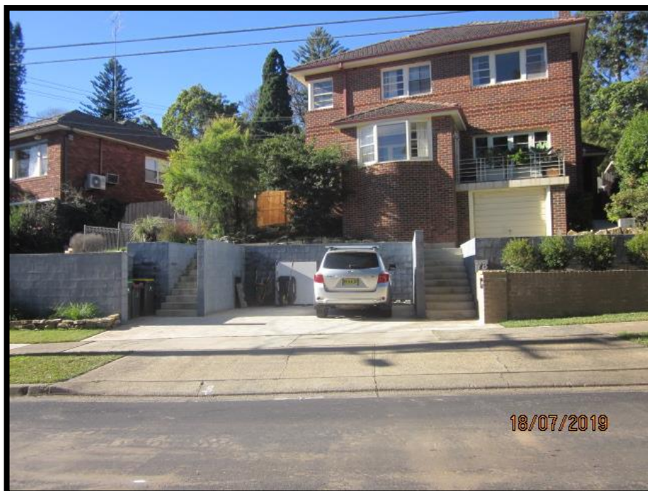
Figure 3: No. 78 East Parade with constructed walls for carport.
