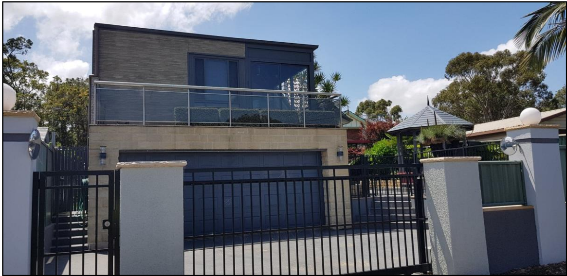
Figure 10: Vehicular access to 14 Norma Avenue.
