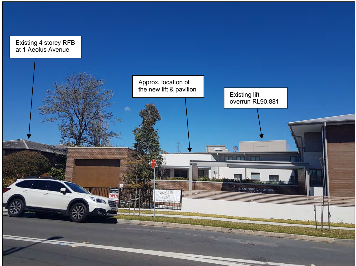
Figure 2 Photo shows the existing building currently occupying the site, viewed from Aeolus Avenue.
