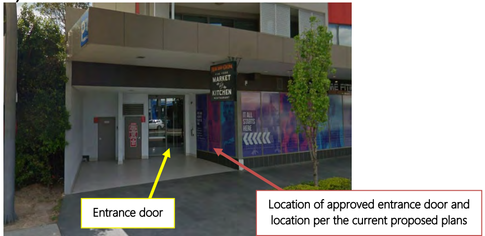
Figure 2. External photograph of the common gym and residents entrance from Victoria Road (Source: Google Street View)
