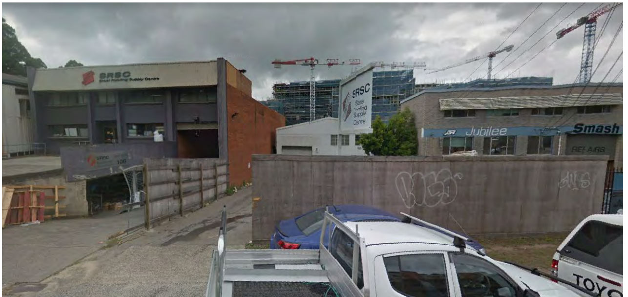
Figure 5: Industrial buildings immediate south of the subject site (106 Bowden Street).
