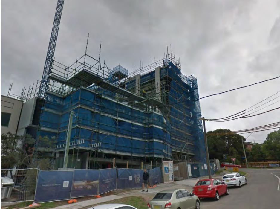
Figure 6: 115 and 117 Bowden Road, opposite the site. 7 storey residential apartment building under construction.
