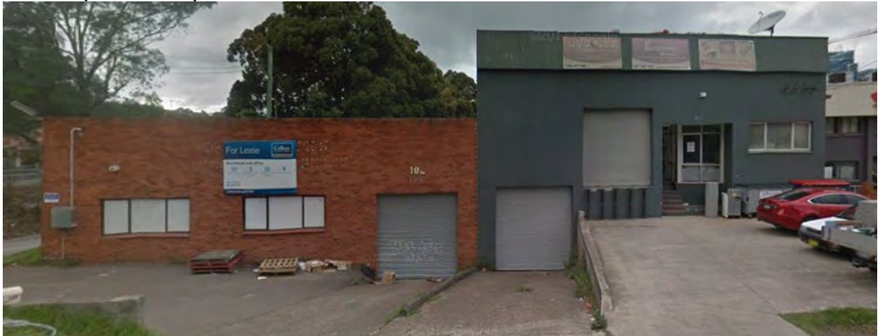
Figure 3: Existing buildings at 102-104 Bowden Street.
