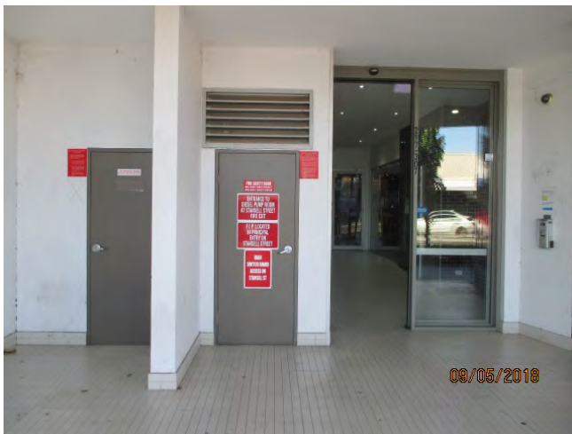
Figure 3. Photograph of front entrance of the gym from Victoria Road (Source: Site Visit 9.5.18)
