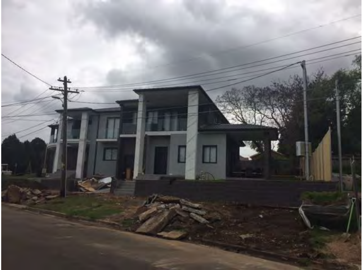
Figure 4. Photograph of subject site under construction – Looking north
