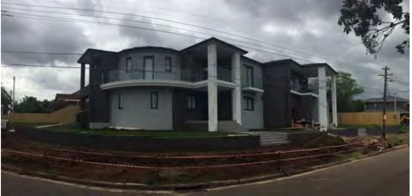
Figure 2. Photograph of subject site under construction – Looking north-east
