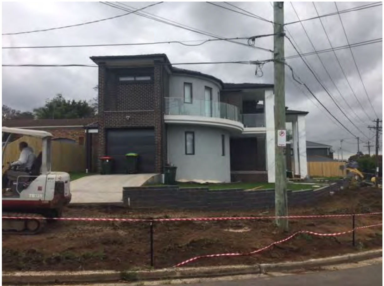
Figure 3. Photograph of subject site under construction – Looking east
