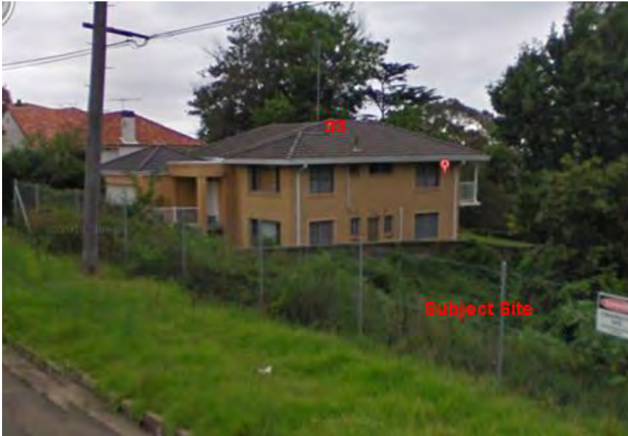
The view from the nature strip looking to No. 33 Wentworth Street
