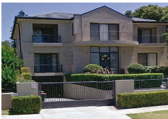
87 Champion Road – two storey above the garage.
