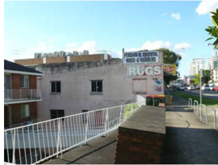
Figure 3: View north to existing building on site.
