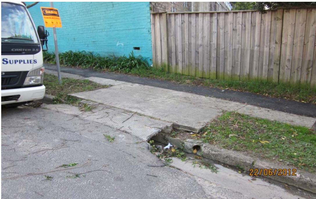
Location of Existing Driveway Crossing (off Cambridge Street)
