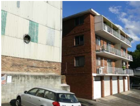
Figure 5: View to neighbouring residential flat building at 31 Devlin Street from Belmore Lane
