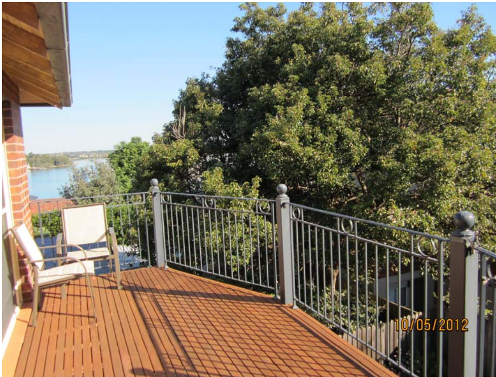
The existing first floor balcony at the rear of the objector's property.
