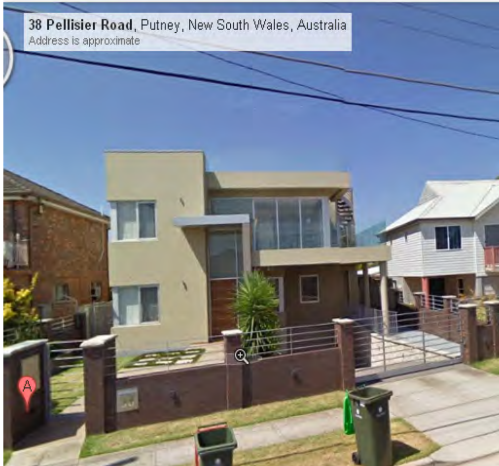
38 Pellisier Road – example of flat roof
