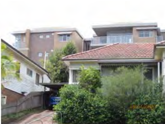
View of part of rear (west) from Samuel St
