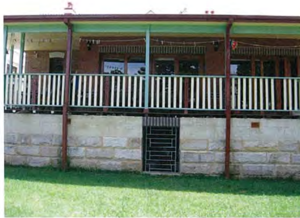
Views of the rear verandah above
