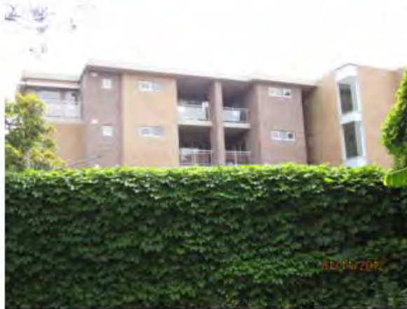
View of rear part of south side from walkway between Blaxland Rd & Samuel St
