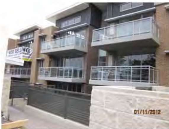
Close up of clear glass facades on Blaxland Rd frontage, all originally approved as solid. Note: air conditioning units are visible
