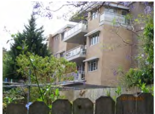
View of part of rear (west) from walkway between Blaxland Rd & Samuel St
