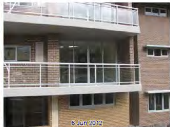
Close up of clear glass facades on northern façade facing fire station, about 40% of each approved as solid
