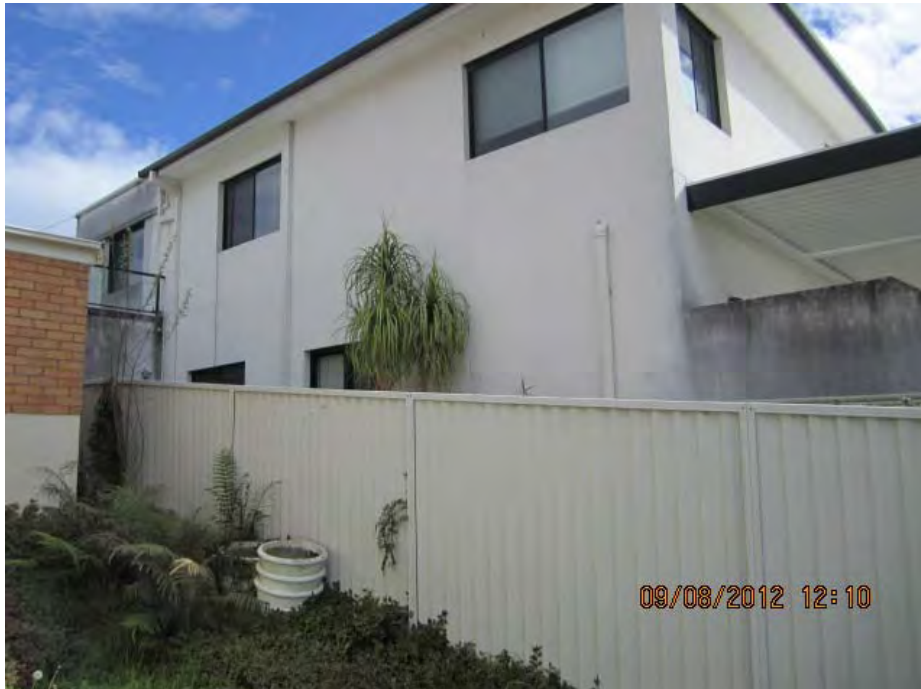
Side windows & rear deck area of 66 Pellisier Road
