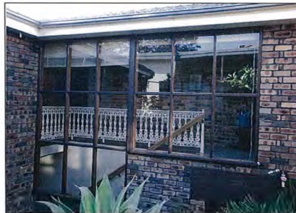
Northern facing windows of 64A Pellisier Road
