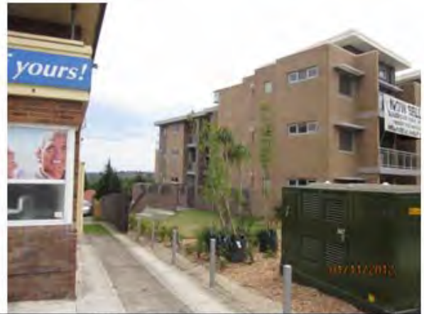
View of south side from Blaxland Rd
