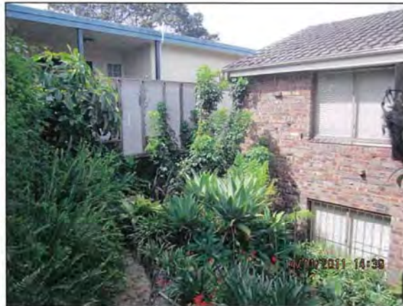
Front courtyard of No. 64A Pellisier Road and west facing windows (note adjoining location of No. 64 Pellisier Road)
