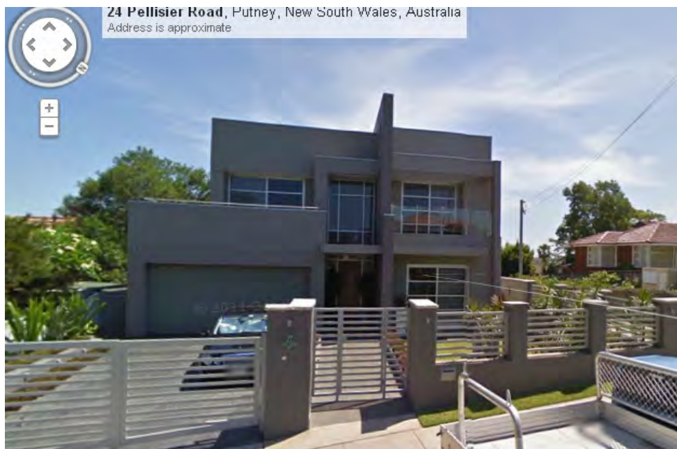
24 Pellisier Road – flat roof and garage at front.
