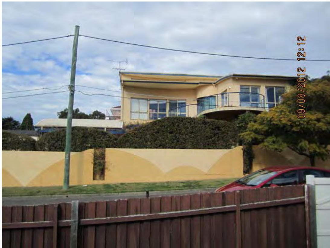
68 Pellisier Road – Streetscape - high solid wall with hedge landscaping along McGowan Street frontage.
