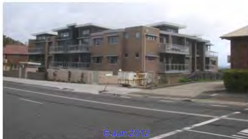
View of clear balustrades on front (east) façade & north (side) façade
