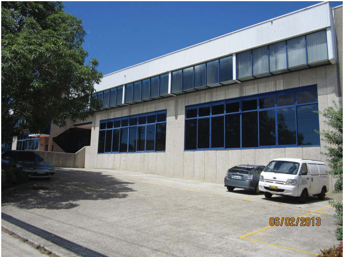
Photo of the western side of the commercial building where gymnasium is proposed
