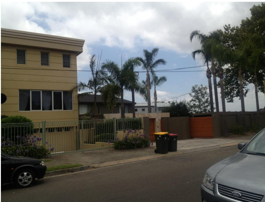
Photograph 2 – Dwelling subject of the proposed alterations and addition to left of frame, with adjoining development at 75A Wharf Road to the right of frame.
