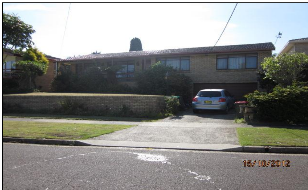
Figure 2: Existing Dwelling (Front Elevation)
