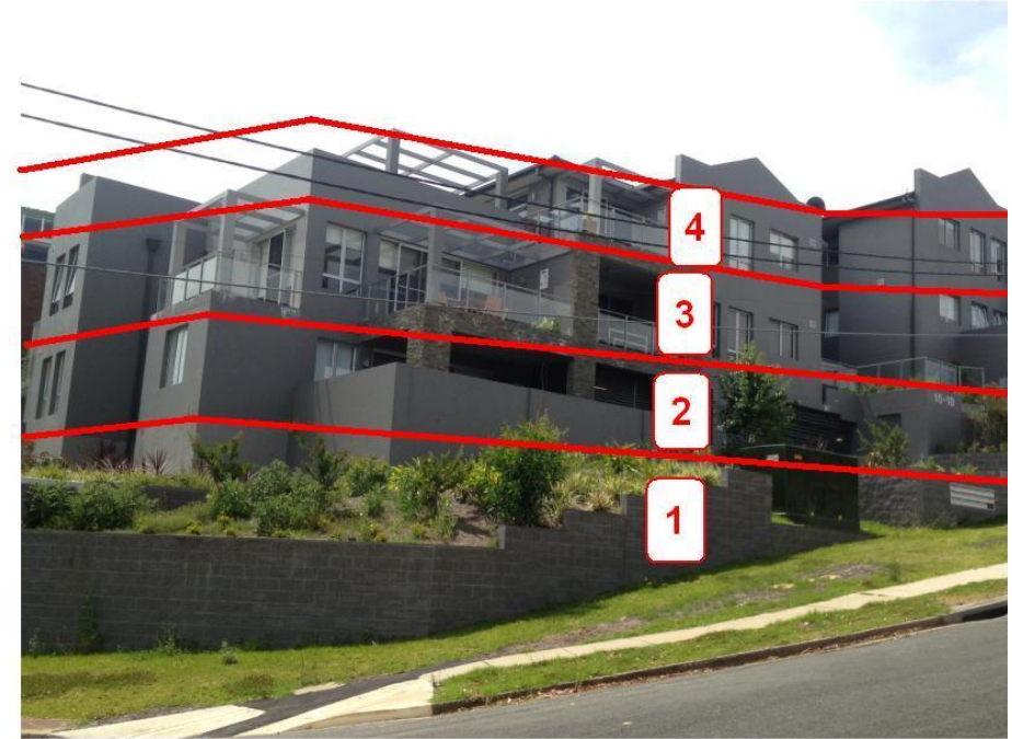
Adjoining subject site to south at 15-19 Gladstone Street, Ryde
