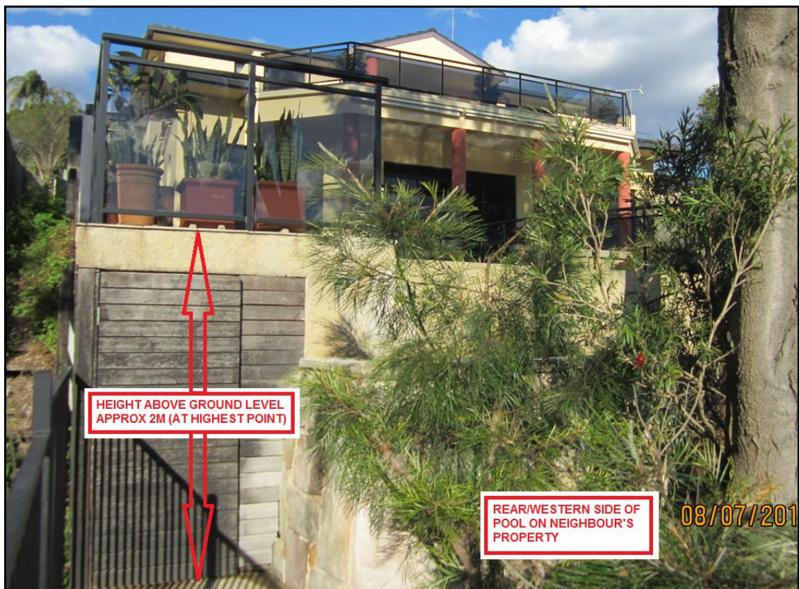
Rear of existing pool on objector's property, showing height above ground level due to topography.
