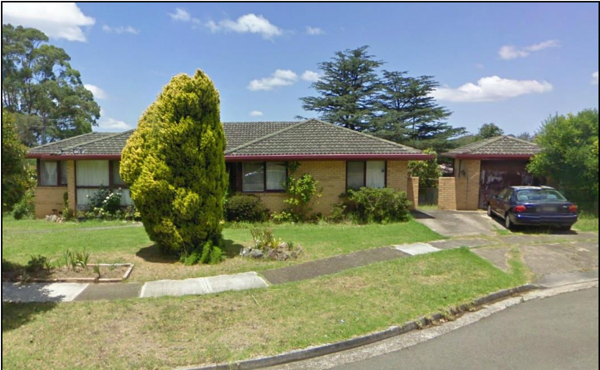
View of subject site from the Coral Street frontage
