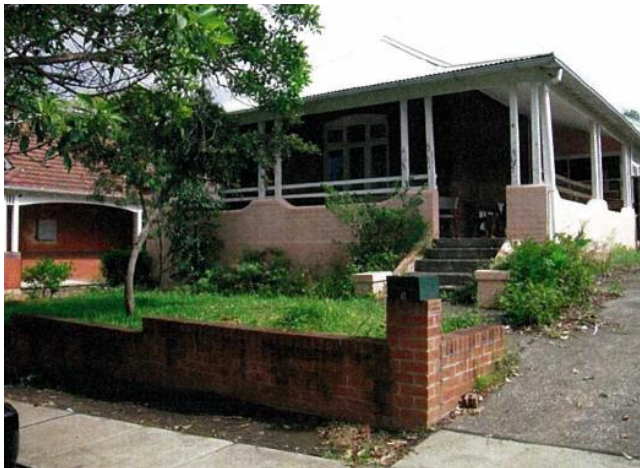
Figure 9: Existing dwelling at 5 Pearson Street – to be demolished.
