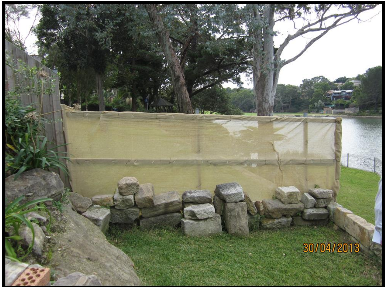
Photo of temporary timber-framed hessian screen
