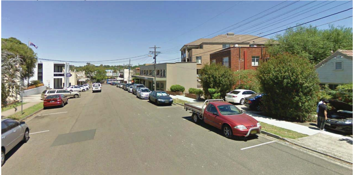
Photo 1: Photo taken from Ethel Street looking west towards the Eastwood Police Station (left), Eastwood Train Station (end of street), two and four storey mixed use development (centre and behind), a two storey office premises (centre) and the existing single storey building on the subject site (right).
