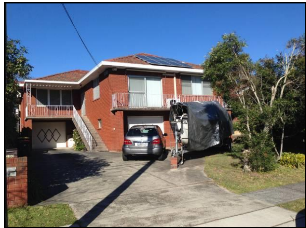
Figure 10 – Raised front porch of existing development on subject site 288 Rowe Street.
