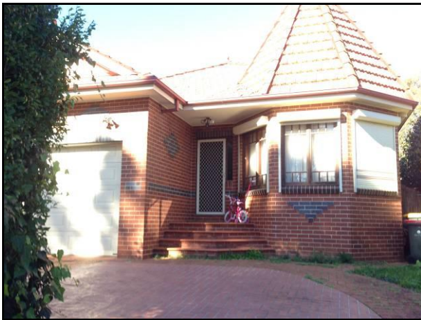
Figure 9 – Raised front porch at 292A Rowe Street consistent with that of the proposed development.
