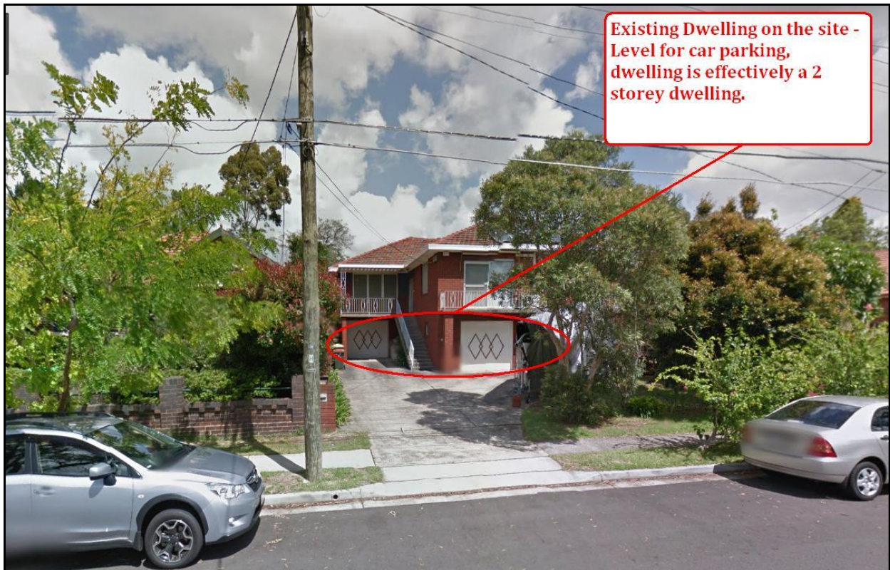
Figure 16 – Photograph of the existing dwelling on the subject site. Indicated is the elevated front porch and balcony on site along with the modified natural topography.
