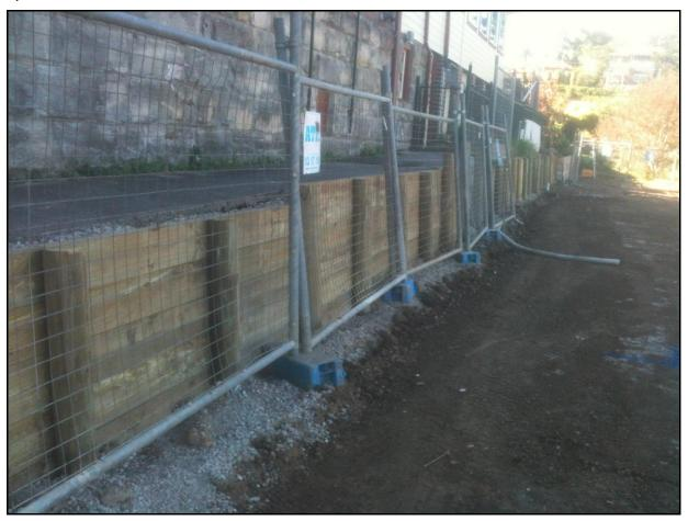
Photo showing the Timber Log Retaining Wall
