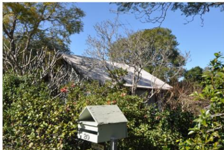
Figure 9: Street view of timber studio structure in north-east corner of site. (Source: Rappoport Pty Ltd, August 2013)
