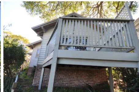
Figure 10: Rear view of timber studio structure in north-east corner of site. (Source: Rappoport Pty Ltd, August 2013)
