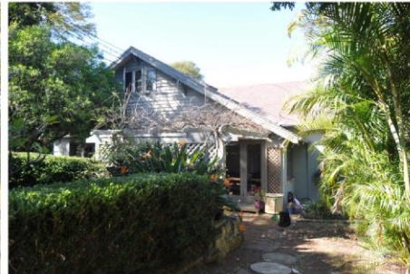
Figure 4: Front façade of existing dwelling. (Source: Rappoport Pty Ltd, August 2013)
