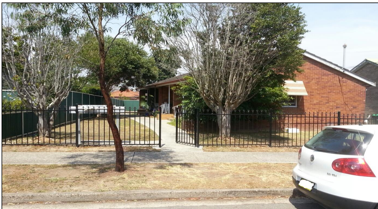
Figure 2: Existing building viewed from Callaghan Street
